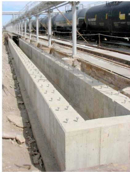
NEW KEMROK Cement Concrete Sulfur Trench
