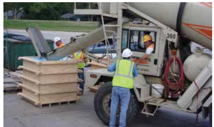
Fig. 2: Concrete placement for a 3 x 3 x 3 ft (0.9 x 0.9 x 0.9 m) specimen
